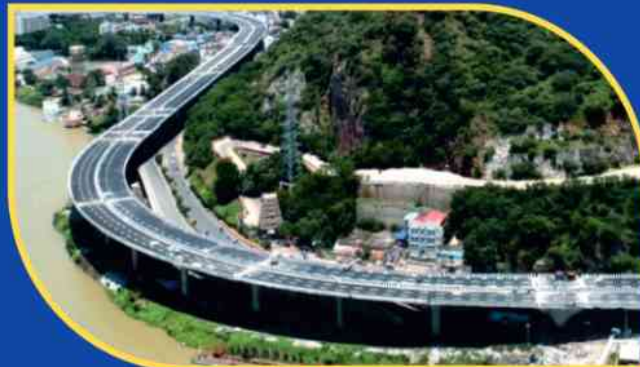
SRI KANAKADURGAMMA FLYOVER
