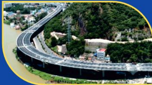
SRI KANAKADURGAMMA FLYOVER
